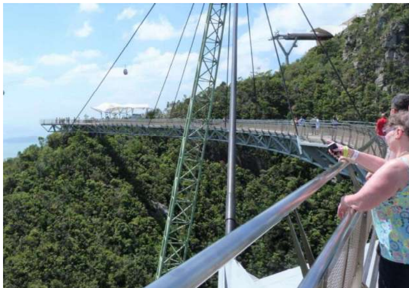
Langkawi Sky Bridge is a 125-metre long cable-stayed bridge in Malaysia, completed in 2005, featuring a curved pedestrian walkway.
